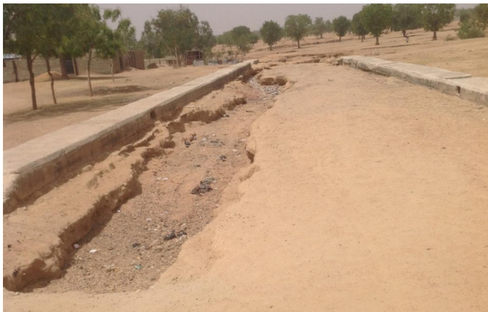
Plate 4: The on-going 5 kilometre road in Dawakin-Tofa town been encroached by gully erosion.
