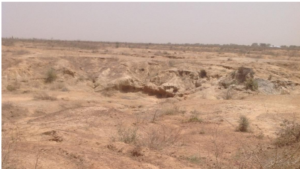
Plate 3: Sections of the Marke steep Gully site Source: Fieldwork, 2017
